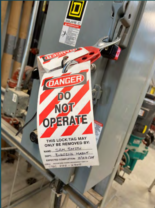
Step 1 – AW removes zip tie and places scissor tag and lock
